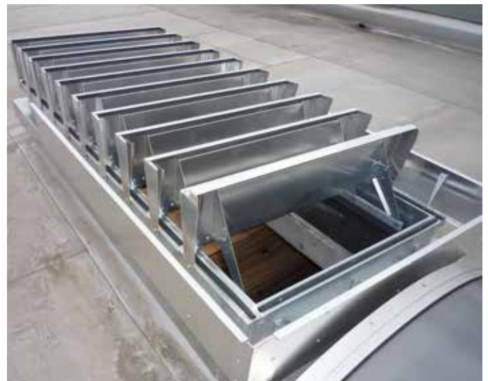
Fig. 40 – mcr LAM louvered vent, roof mounted
